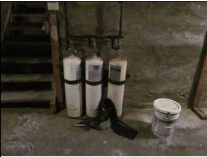
81. View of the kitchen fire retardant system in the kitchen basement.
