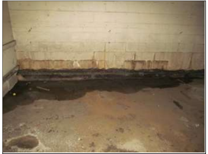
56. View of water seepage inside the golf cart storage building.
