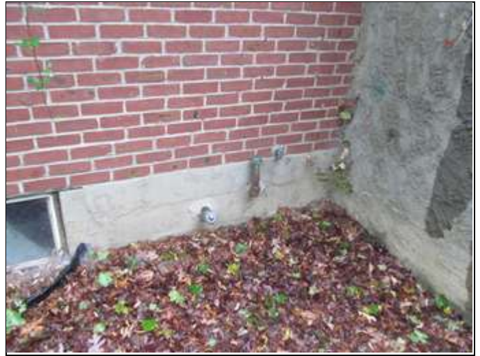
26. View of the fill port and vent pipe at 450 Lakeland Avenue.
