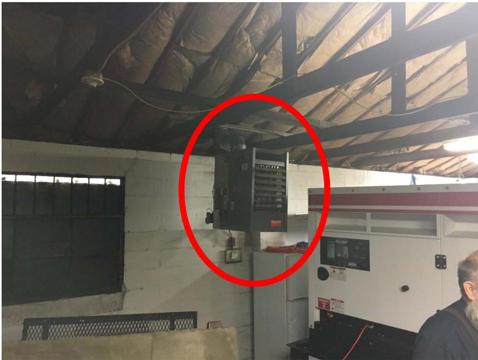
A gas-powered HVAC Air Handler located in the SMB.
