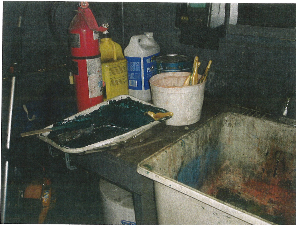
Photo 7 –View of the slop sink in the garage building. Evidence of chemical dumping was evident by the condition of the sink.
