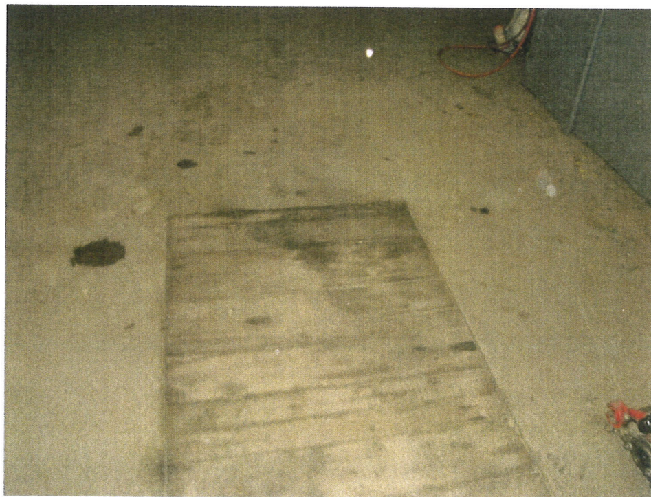
Photo 6 – View of the old repair pit observed in the garage building.
