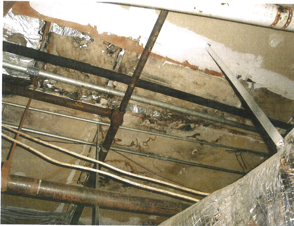
Photo 9 – Water damage and possible mold growth which was observed in the clubhouse building.
